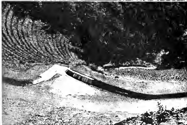
FIGURE 11. Top—Debris spillway entrance on rock slope in foreground. Bottom—Lined debris spillway entrance. Upper right—Typical debris basin spillway in mountainous terrain, lined spillway in background and unlined spillway in foreground
